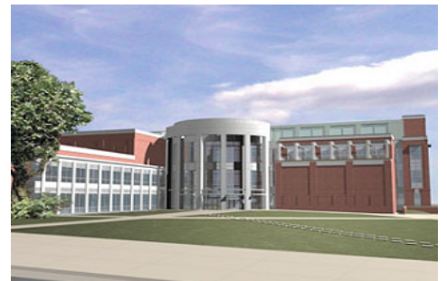
The new Jeong H. Kim Engineering Building will open in 2005.
